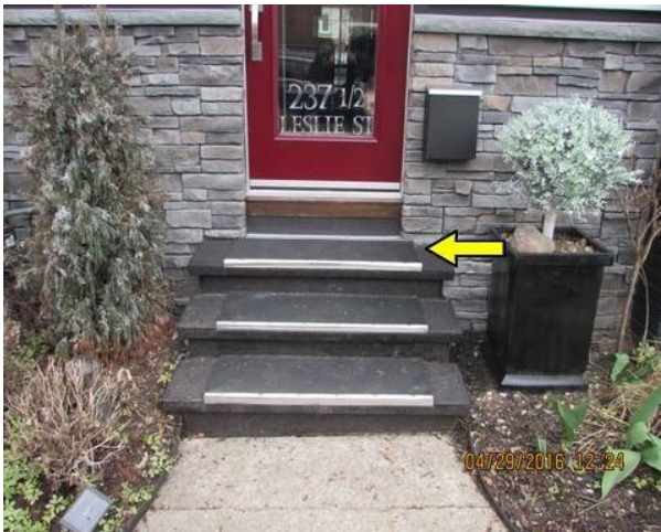
Missing handrail
